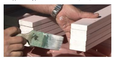
Photo 2: Also apply oil-based alkyd primer over supplementary preservative applied to all cut ends, holes, notches etc
