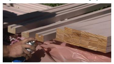
Photo 1: Avoid premature failure by applying a brush on or spray on supplementary preservative to all cut ends, holes, notches etc.
