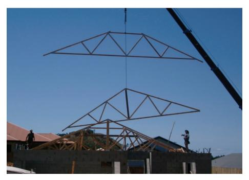
Photograph 3 - Incorrect lifting of trusses
