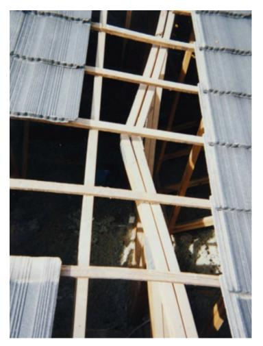
Photograph 5 – Inadequately fixed roof battens resulting in lateral buckling failure of girder truss
