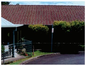
Photograph 6 – Distorted rows of roof tiles and trusses due to inadequate roof bracing
