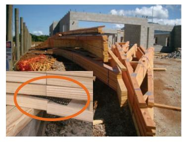
Photograph 1 - Don't install site damaged trusses or those with manufacturing faults. Replace or repair before erecting
