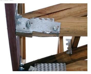
Photograph 7 - Girder brackets not installed correctly
