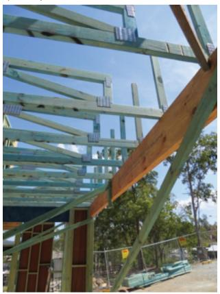
Photograph 11 - Structurally deficient parapets
