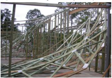
Photograph 4 – Dangers of not providing temporary bracing
