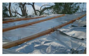
Photograph 5 – Roof sheeting and battens have failed due to nailed batten fixing where screws should have been used
