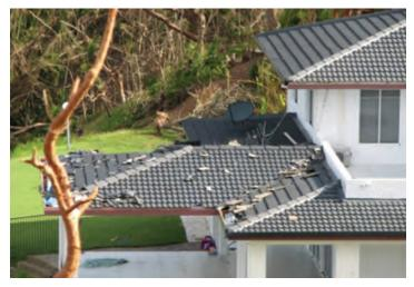
Photograph 3 – Inadequately fixed tiles dislodged after high wind event
