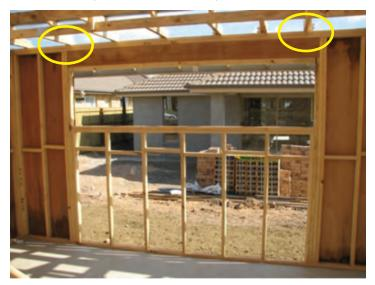
Photograph 11 – Plywood cannot be used to effect tie-down at sides of openings as the trusses highlighted above must have 300 mm min of ply to the right and left side respectively
