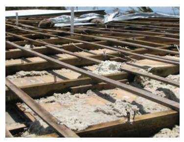
Photograph 4 – Roof sheeting 'blown' off due to inadequate fixing of the sheeting to the battens
