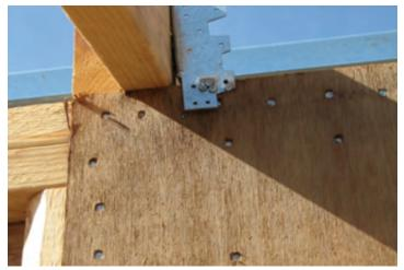
Photograph 2 – A structurally inadequate and incorrectly installed multi-grip. Nails too close to each other and edge of metal and also, too close to top edge of top plate
