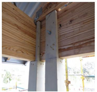
Photograph 14 – Posts over checked, bolted connection would not achieve any tie-down capacity
