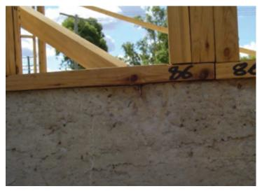
Photograph 13 – Nominal bottom plate connection compromised by excessive plate overhang
