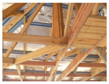
Photograph 8 – Inadequate connection of jack and hip trusses to girder truss for a C2 wind classification
