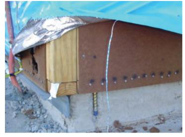
Photograph 12 – Structural integrity totally compromised by excessive bottom plate overhangs
