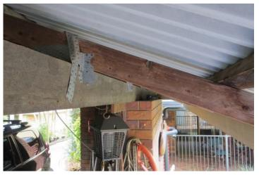
Photograph 1 - ACCEPTABLE – Z275 bracing, multigrips and truss plates in a Low Hazard (>10km from surf) Sheltered Condition. Note: Connectors have been installed for 35 years.
