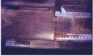
Photograph 3 - NOT ACCEPTABLE - Z275 connectors in deck joists 1 km from surf. 6 years old, Sunshine Coast.
