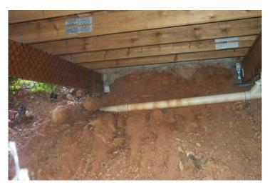
Photograph 4 - NOT ACCEPTABLE – Uncoated Z275 nail plates and framing anchors in Low Hazard Zone but Exposed Condition under a deck.
